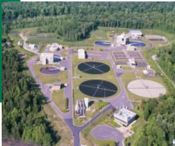
Overview of Rock Hill Waste Water Treatment Facility
